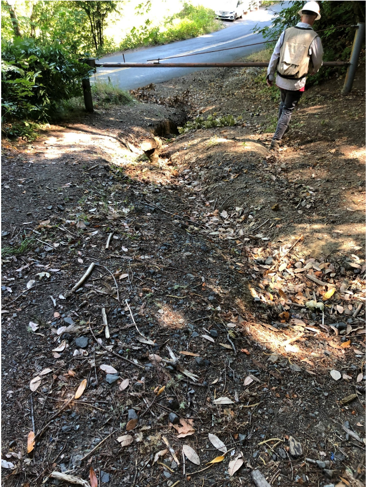
Figure 3. Gully erosion caused by overtopping of inlet pool at Map Point 1.
